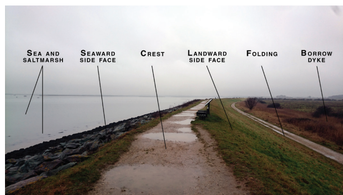
Fig. 1. The typical composition of a sea wall (Brightlingsea, Essex); credit K. Fargeaud.
